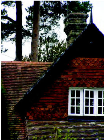
Picture 9.17 Gable ends
