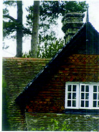
Picture 9.17 Gable ends
