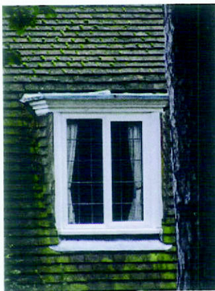
Picture 9.39 Box windows
