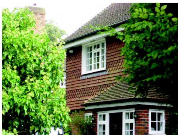
Picture 9.13 Tile hanging
