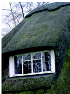
Picture 9.31 Thatch roof
