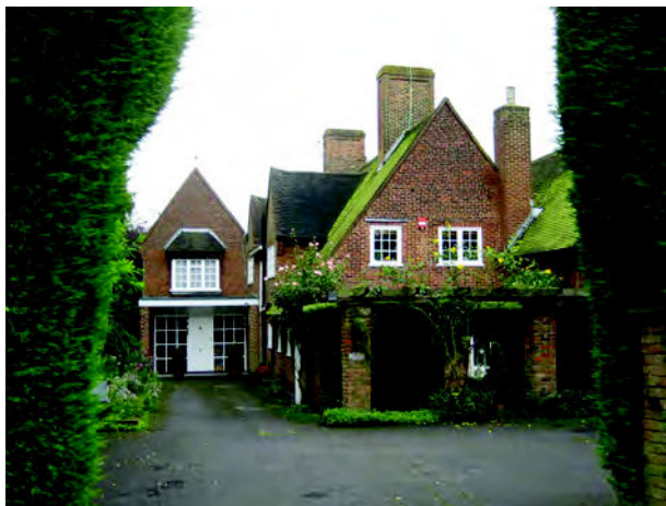
Picture 9.19 Steeply pitched roofs
