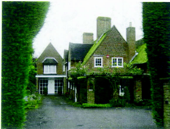
Picture 9.19 Steeply pitched roofs
