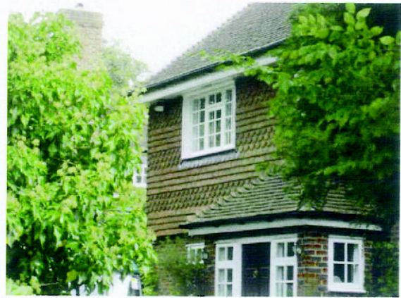
Picture 9.13 Tile hanging
