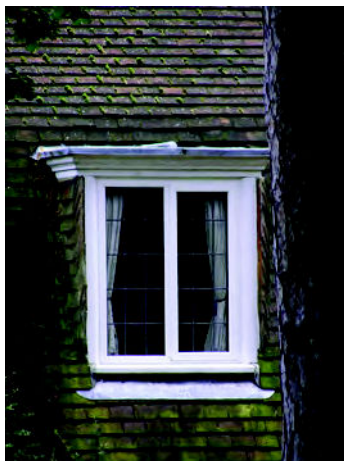
Picture 9.39 Box windows
