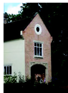
Picture 9.27 Stone lintels
