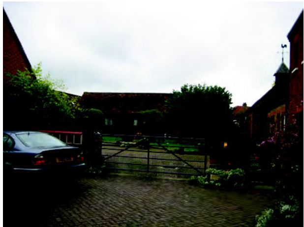
Picture 9.46 Farmyard gates
