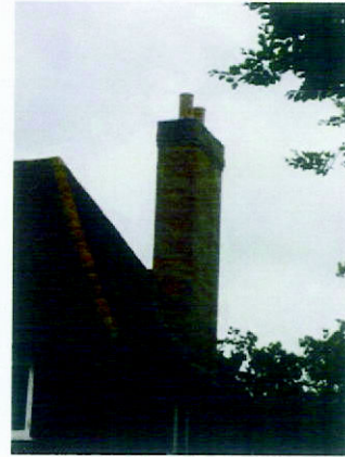
Picture 9.18 Tall chimneys
