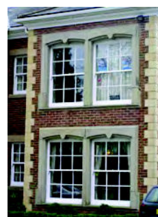
Picture 9.36 Stone quoins and window surrounds
