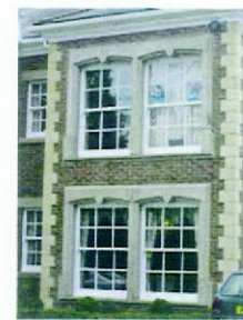
Picture 9.36 Stone quoins and window surrounds
