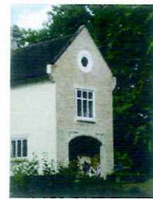
Picture 9.27 Stone lintels
